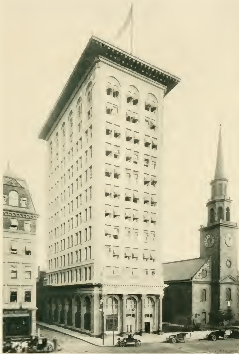
NATIONAL STATE BANK, BROAD AND MECHANIC STREETS.
